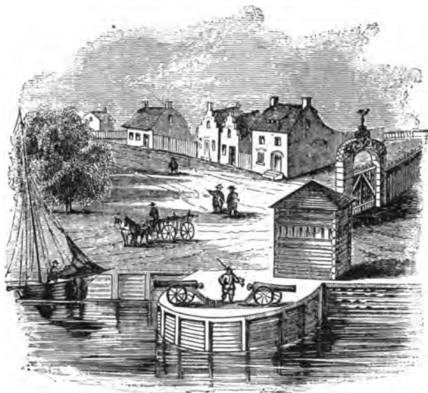
THE WATER GATE.
